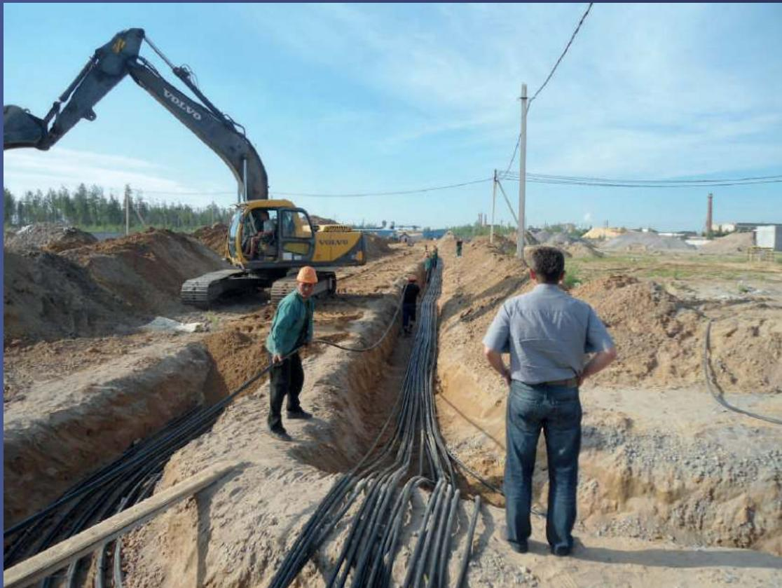
Integrated engineering and implementation work construction of FOCL «turnkey» for connection of objects in Atyrau region to telecommunications network «Transtelecom»
