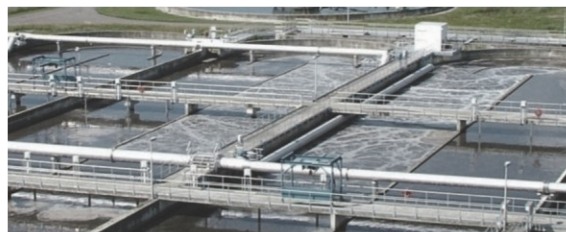
CASPIAN CONTRACTORS TRUST
