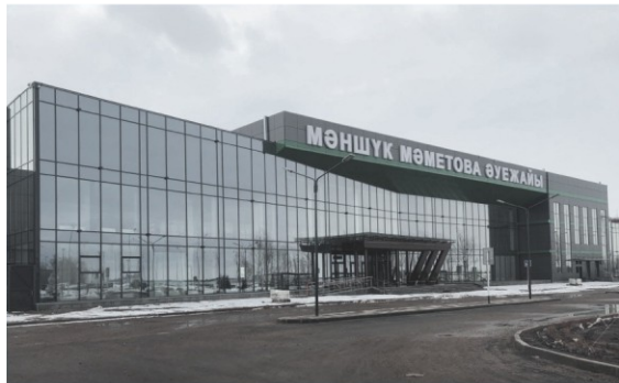
RECONSTRUCTION OF THE BUILDING URALSK CITY AIRPORT
